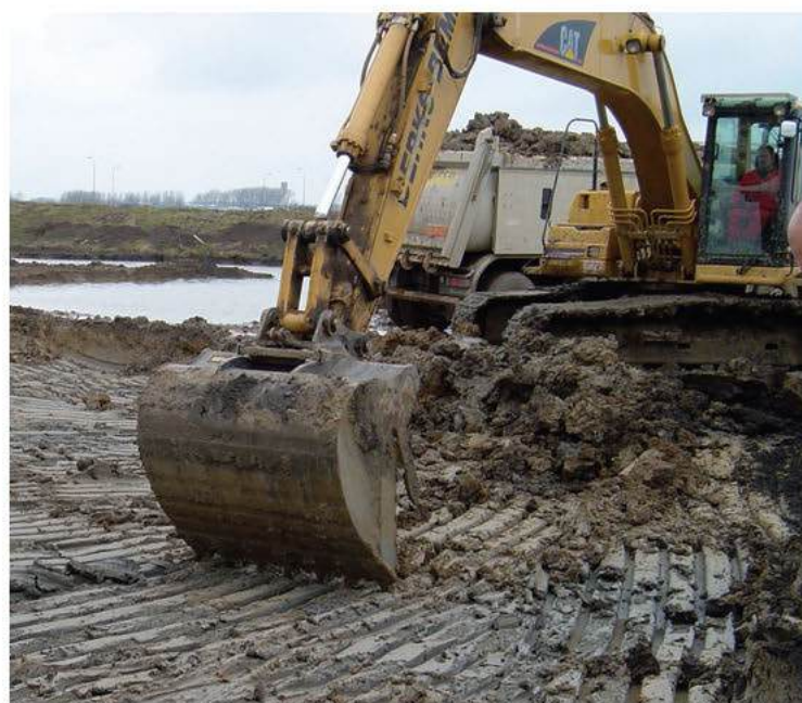
Fig. 6. Left panel: the extraction of clay using a backhoe, near the town of Arnhem (Fig. 2). Right panel: the extraction depth is about 1 m (including ~30 cm of overburden); relevant lithological variation on that vertical scale is clearly visible. A caliche-horizon within the oxidised clays (not visible on this scale) presents a challenge, as it has to be removed before continuing extraction. Photo: DM.
