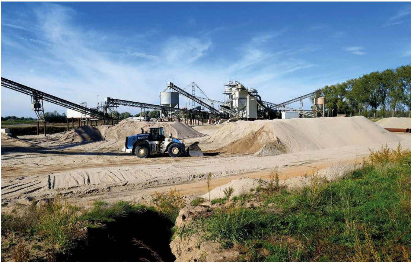
Figure 18.20. Aggregates classification plant near Gendt, Netherlands. Photo by Rudolf Bak.
